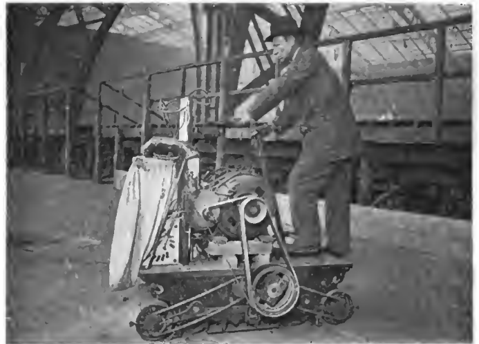
AMERICAN OPERATOR AND MACHINE PLANING PARIS TRACKS.
